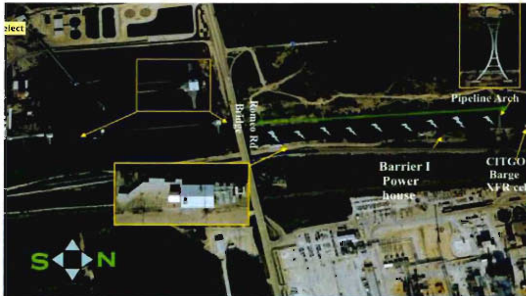
Figure 1: Aerial view of the Chicago Sanitary and Ship Canal Aquatic Nuisance Species Dispersal Barrier (“Barrier I”), located in Romeoville, IL (Source: U. S. Army Corps of Engineers, Chicago District)
